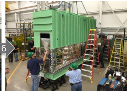
Vessel cover installation
