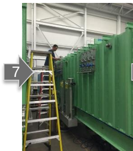
Tuner valve manifold installation
