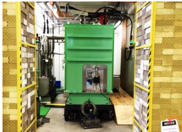
Bunker test system
